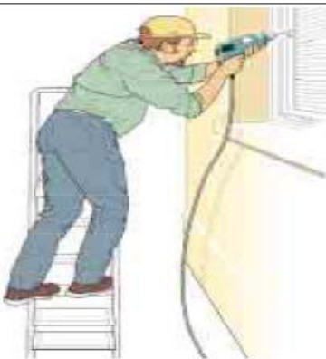
Correct – two clear rungs. Don't work any higher up this type of stepladder.
